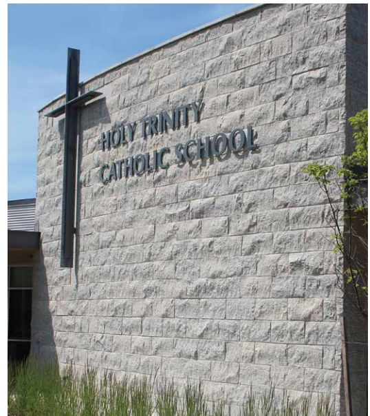
Holy Trinity Catholic School - Sarnia, ON; Architect: Randy Wilson Architect Inc. of London; Product: Masonry Units; Color: Blue Grey Veined; Finish: Fine Dressed and Split Face
