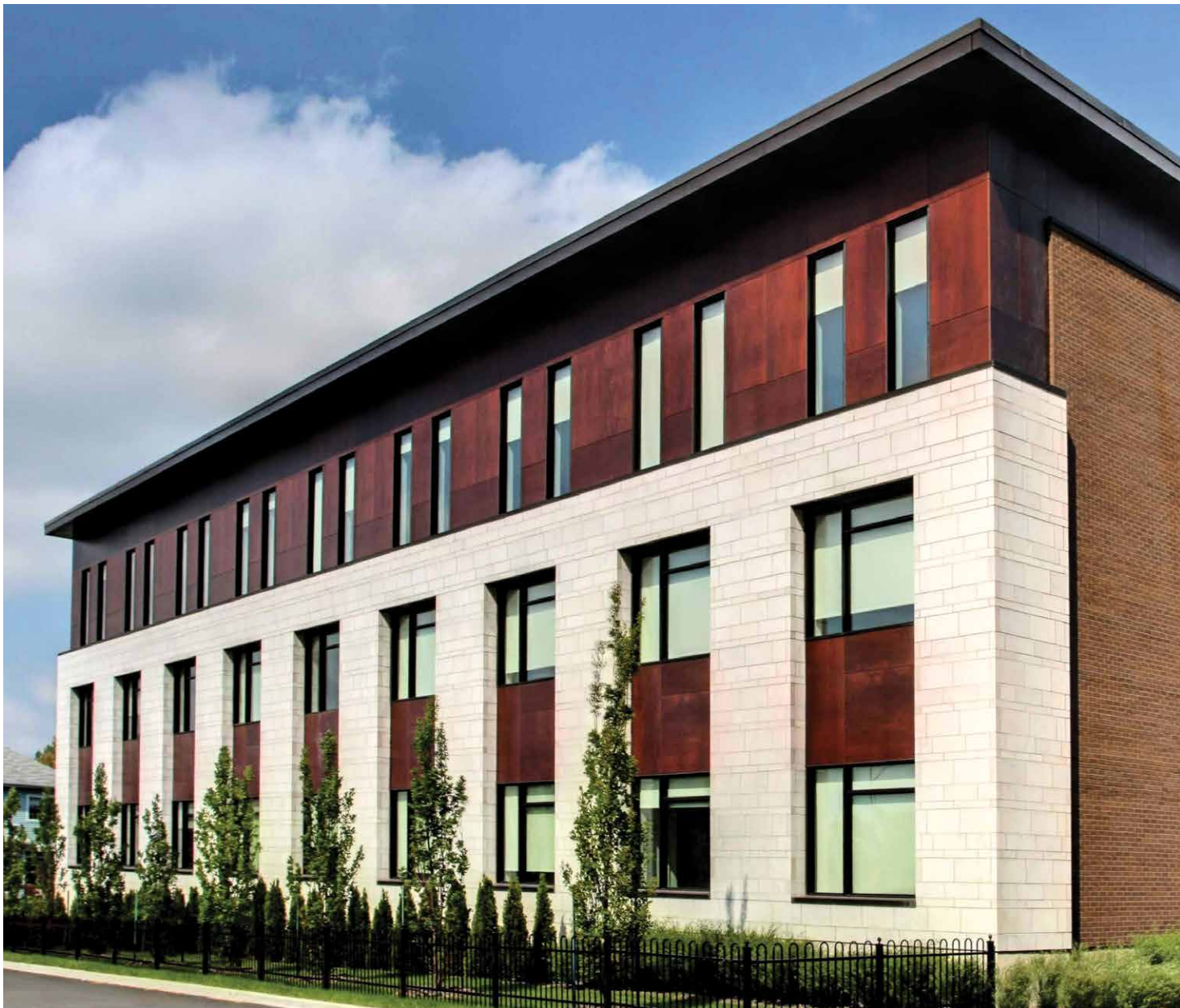
Ronald McDonald House, Montreal, QC; Architect: Manon Renaud Architect; Product: Masonry Units; Color: Sepia Fleuri; Finish: Medium Dressed
