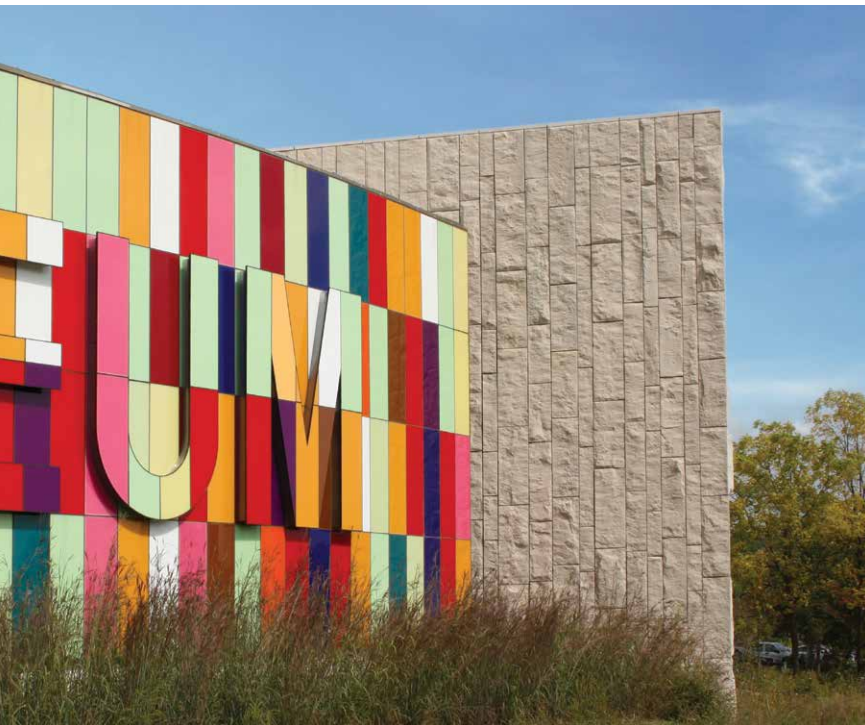
ON; Architects: Moriyama & Teshima Architects, The Walter Fedy Partnership; Sepia; Finish: Split Face
