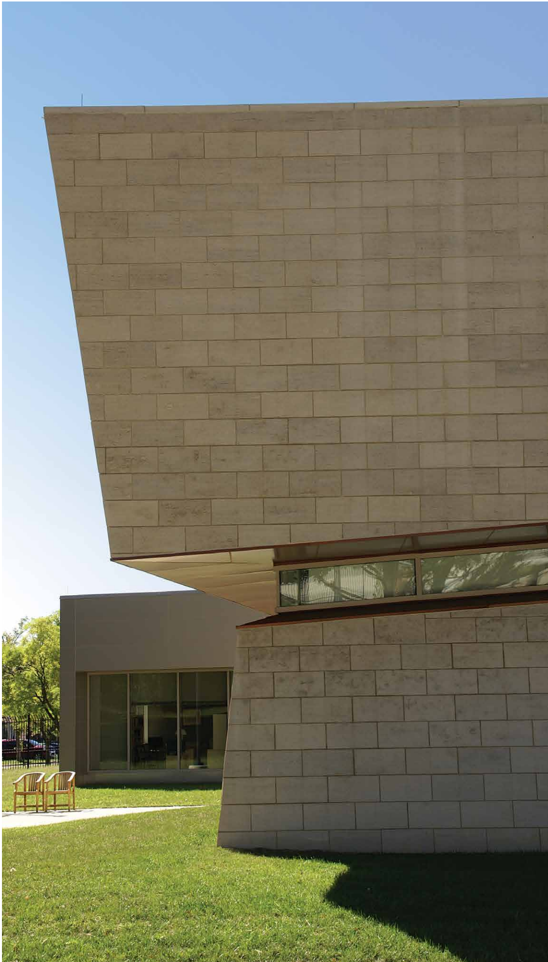
National Museum of Health and Medicine, Silver Spring, MD; Architect: KlingStubbins; Product: Masonry Units; Color: Sepia Veined; Finish: Fine Dressed
